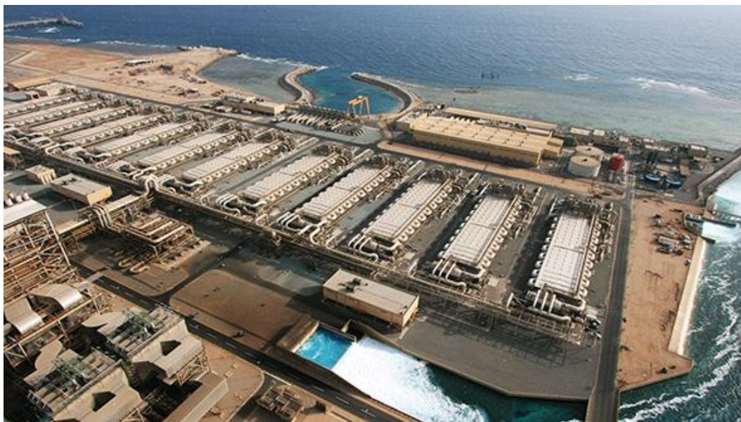
Figura 1.2 Usina de Ras Al-Khair
